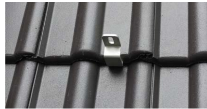
Figure 5 (EJOT® Solar Hook Installed)
