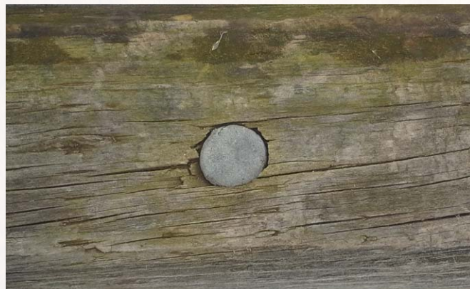
Figure 3: Hot Dipped Galvanized Fastener Example in Treated Landscape Timber after Several Years Exposure 图3、热镀锌紧固件暴露于处理的景观木材数年后的实例
